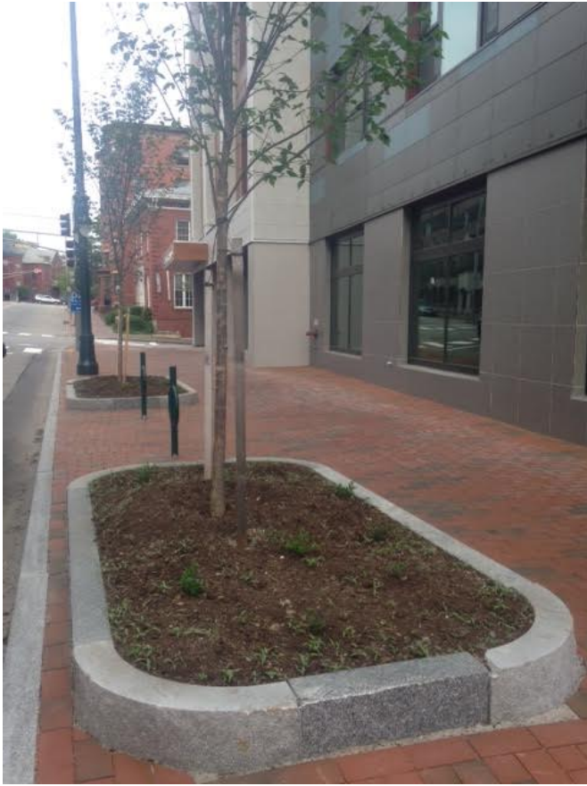
Portland planter standard with either 1' or 2' radius corners depending on size.
