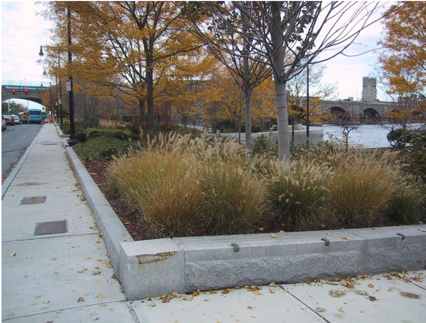
Boston Rose Kennedy parkway granite planter seatwall with anti skateboard blocks
